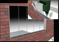
Set out dry the first row of glass blocks to ensure opening size is correct. Mark accurately and drill oversized holes in between the blocks, vertically and horizontally where rods will be positioned. Fill holes with silicone and fit vertical bars in place.
