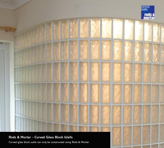
Planning the design of a curved wall uses the same principles of constructing a flat wall. Additional considerations to address are calculating the opening size, ensuring the internal radius is sufficient in respect of the block size being used and positioning of intermediate vertical slip joints.
