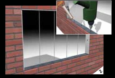
Set out dry the first row of glass blocks to ensure opening size is correct. Mark accurately and drill oversized holes in between the blocks, vertically and horizontally where rods will be positioned. Fill holes with silicone and fit vertical bars in place.
