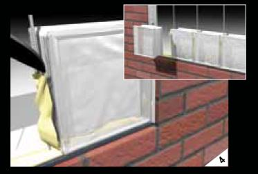
Fit first block and tamp down gently, fit second block and repeat. Ensure there is enough mortar between the blocks and the base to create sufficient adhesion, compact the vertical mortar joint using a wooden instrument. Spacer pegs are required between base and first row of blocks.
