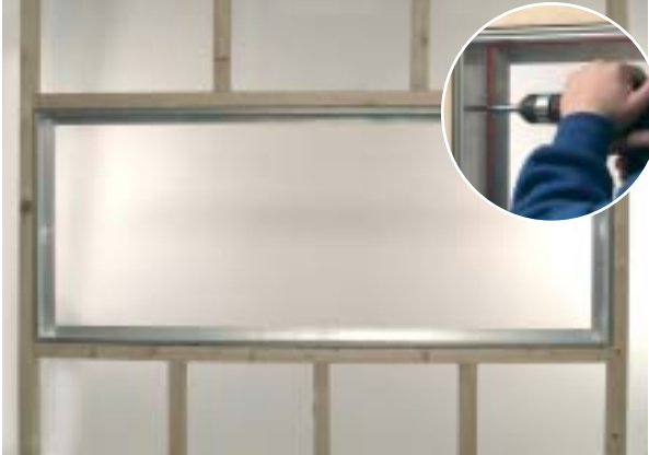
Step 1 : Position and screw in place first part of aluminium channel. Ensure that the screws are located to the relevant marker.
