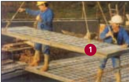
Floor panel being craned into position.
