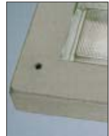
Panel showing location of lifting socket
