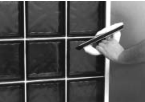
Grouting with Colmef Vetromix glass block mortar
